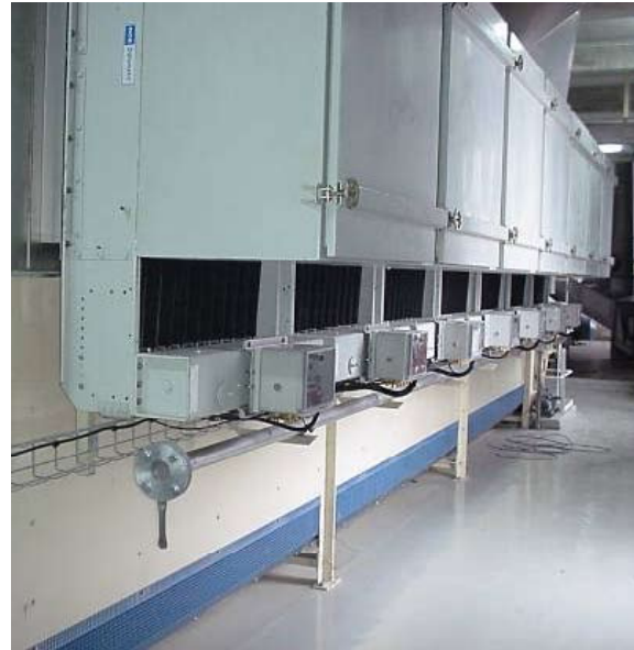
2 passages cooler fitted with filters
