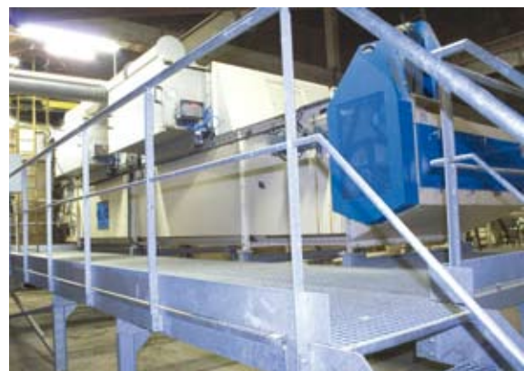
2 passages cooler fitted with filters
