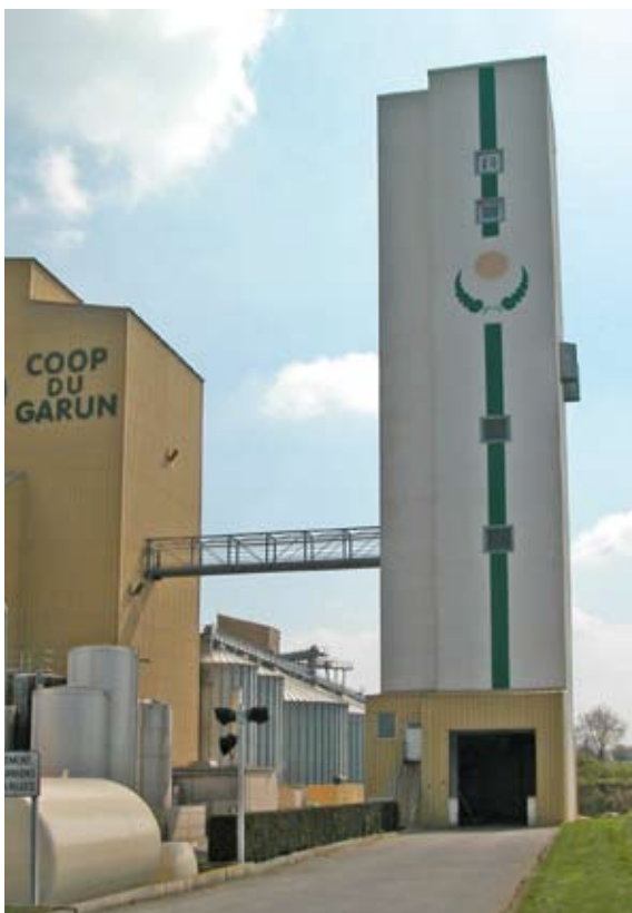
Heat treatment tower «Coop du Garun, France» fully isolated for non contamination.
