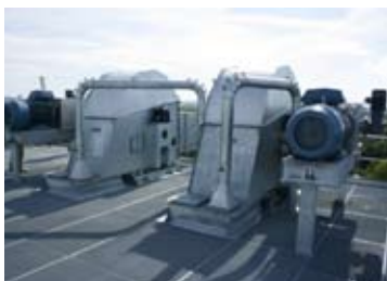
Elevators with discharge suction intakes
